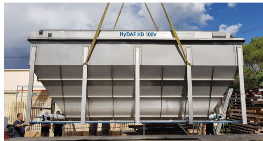
Standard HD-100 model being installed to remove metals from ground water following completion of major tunnelling project in NSW.
